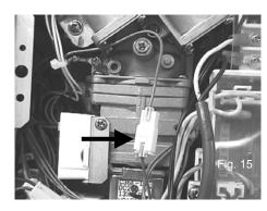
Remove (1) screw from the bottom cable support bracket and fit the white cable support supplied. Pass the cable tie through the loops and around the Communication Cable C. (Fig 16).
