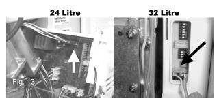
6). For the 32 only locate the 2-pin connector on the Infinity wiring loom and remove the blanking plug. (Fig 14).
