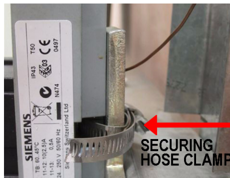
Figure 37 - Securing Hose Clamp
