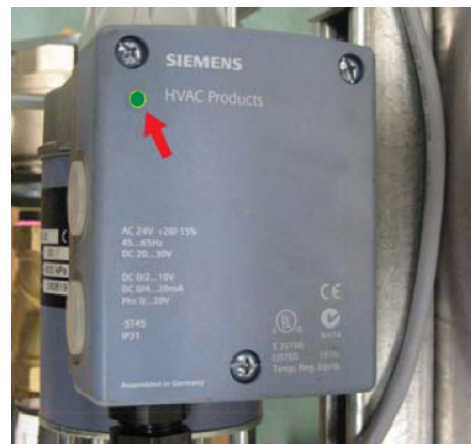
Figure 12 - Power Supply to Control Valve Actuator Controller
