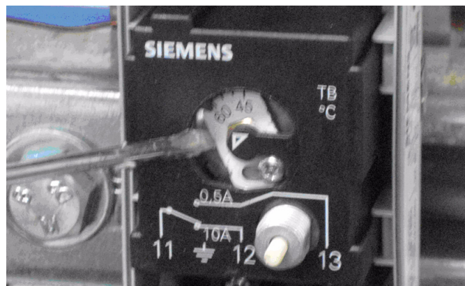
Figure 23 - Rotate Limit Thermostat Switch
