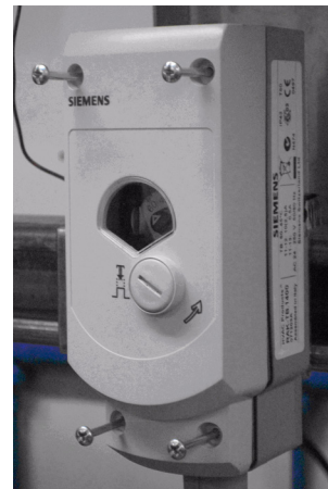
Figure 21 - Removal of Front Cover
