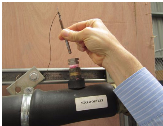
Figure 13 - Removal of Limit Thermostat Probe
