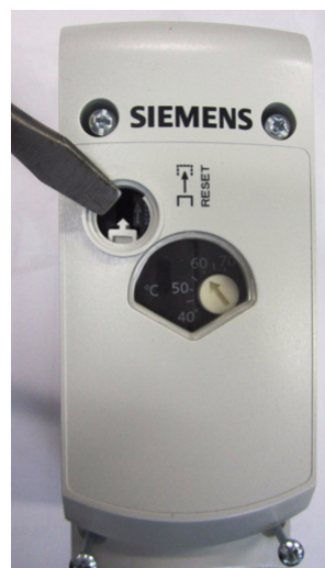
Figure 15a - Resetting Limit Thermostat
