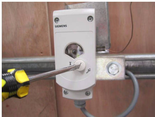
Figure 14 - Remove of Access Cover
