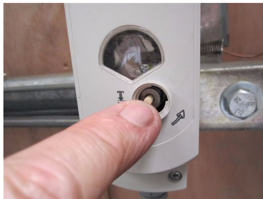
Figure 15 - Resetting Limit Thermostat
