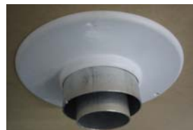
"TOP" marking on BOTTOM of plastic spacer (through wall vertical co-axial installation only).
